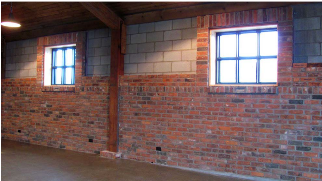
Interior view of the east wall showing exposed sections of the east wall that had to be rebuilt with concrete block after a “freak accident”. On the morning of December 8, 2000, a dump truck had a break failure while travelling down the very steep Sydenham Hill. The truck safely rolled through the intersection at King Street, veered into the parking lot on the east side of the warehouse and crashed through the brick masonry wall ( https://www.lagershed.com/our-story ) of the Valley City warehouse.
