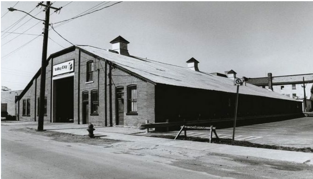
Circa 1981 photo of the Valley City Manufacturing Co., after the piers flanking the rolling door had been cut back to the roofline and the original skylights covered (likely at some point when the building was re-roofed). By this time two of the window openings on the east side of the rolling door had been replaced by two doorways, possibly when the building was converted to a bus depot. All other windows are still the original two-over-two paned wood sash ones. (Dale Creasy, unused photo for the Picturesque Dundas Update – 1981 , DM&A)
