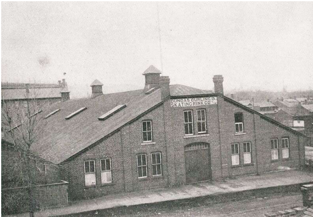
The Dundas Curling & Skating Rink, circa 1896. Photo shows the original façade with a single carriage entrance, and the original windows, four of the eight skylights and three square roof vents. ( Picturesque Dundas – 1972; reprint of original 1896 publication. (Dundas Museum & Archives: DM&A)
