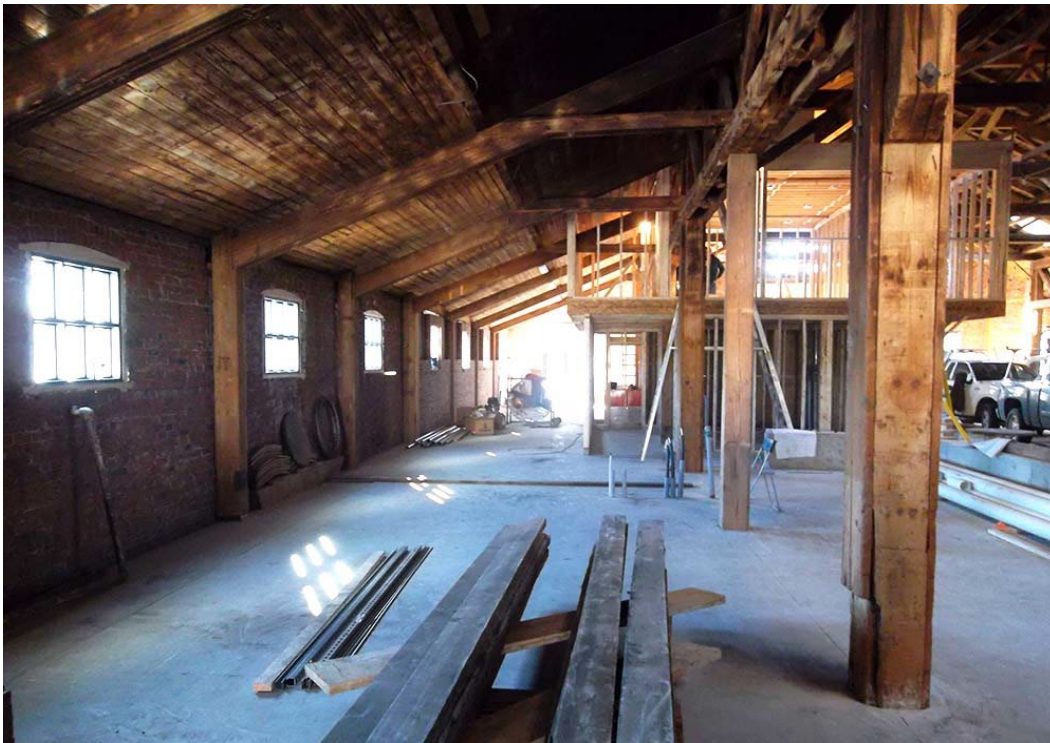
View of the interior while still under construction in January 2016, looking towards the front entrance and showing the east wall rebuilt with concrete block, as explained below. The framed mezzanine level was intended to provide office space with washrooms on the ground floor. (Jeremy Parsons)
