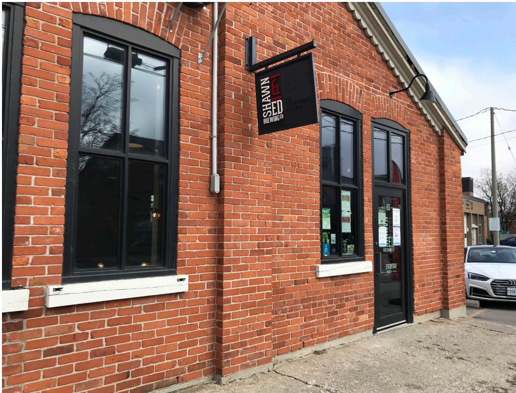
Close-up view showing the replacement steel windows with a two-over-two configuration replicating the original wood sash windows and shaped to fit the voussoir-arched brick lintels.
