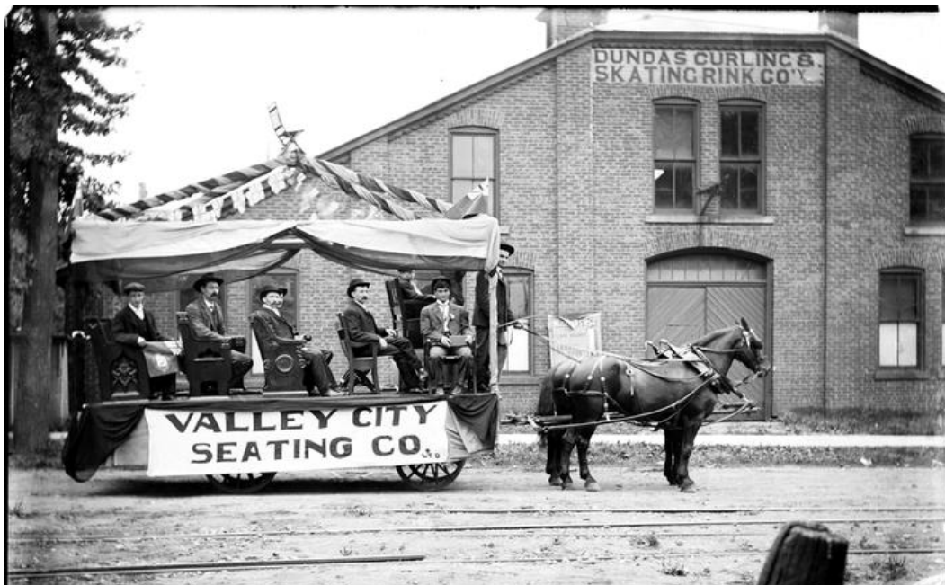
A horse-drawn parade float for the Valley City Seating Co. in front of the Dundas Curling & Skating Rink, circa 1910. Shows the double diagonal board doors of the carriage entrance with a voussoir-arched brick lintel and transom light. (DM&A: GN-0346 - cropped)
